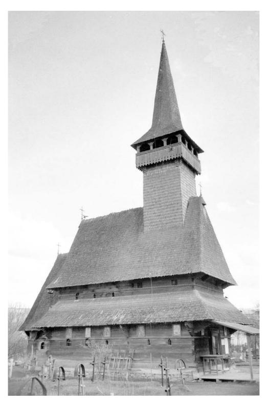
Sat Şugătag. The church is preserved in good condition. One of the specific features is the mouldings surrounding the log fabric on two levels, above both rows of windows. Wherever the horizontal mouldings appear they are cut above apertures indicating a symbolical distinction between the earthly world and the one above. Photo: April 1994.
