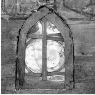
wooden nails into a groove following the aperture in the wall. The bottle glasses, for the most part used in small shivers, were embedded in the frame by delicate grooved pieces of sycamore maple wood. Until the end of the 18th century, the majority of the churches were supplied with such windows.
