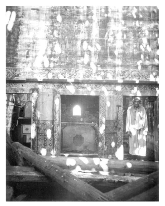
**8** *Berbeşti*. Photo by Atanasie Popa, July 1932, just before its demolition (MIT, Arhiva CMIT, C3:4778). The picture was taken from inside the nave looking towards the sanctuary. The spots of light on the iconostasis and the timbers lying on the floor indicate the roof was in a poor state and the vault had fallen in.
