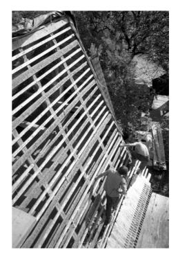
**94** *Ieud Deal.* The old lathing was easily distinguishable by its massive appearance under the repair of the roof. Photo: August 1997.
