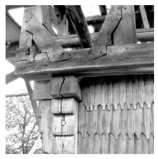
**133** *Deseşti*. During the repairs from 1996, the hidden parts of the tower were exposed revealing numerous assembly marks of great variety. Here there can be observed the graphic signs "+" and "III" on both the gallery posts and their respective downward angle ties. Unfortunately, some of them were lost with the replacement of some original pieces and some due to the "cleaning" of the surface with an axe without any thought for their historical value. Photo: June 1996.
