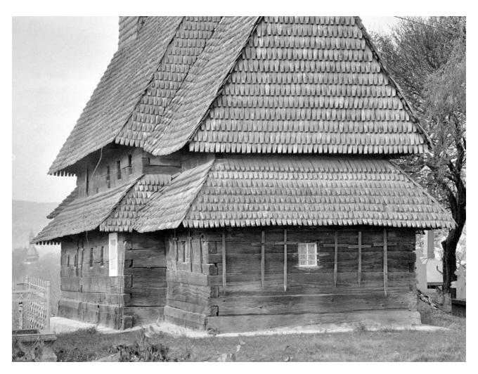
**45** *Apşa de Mijloc Susani.* This medium sized wooden church, from the first decade of the 18th century, was excellently built with well levelled walls and flush covert joints. Photo: October 2000.
