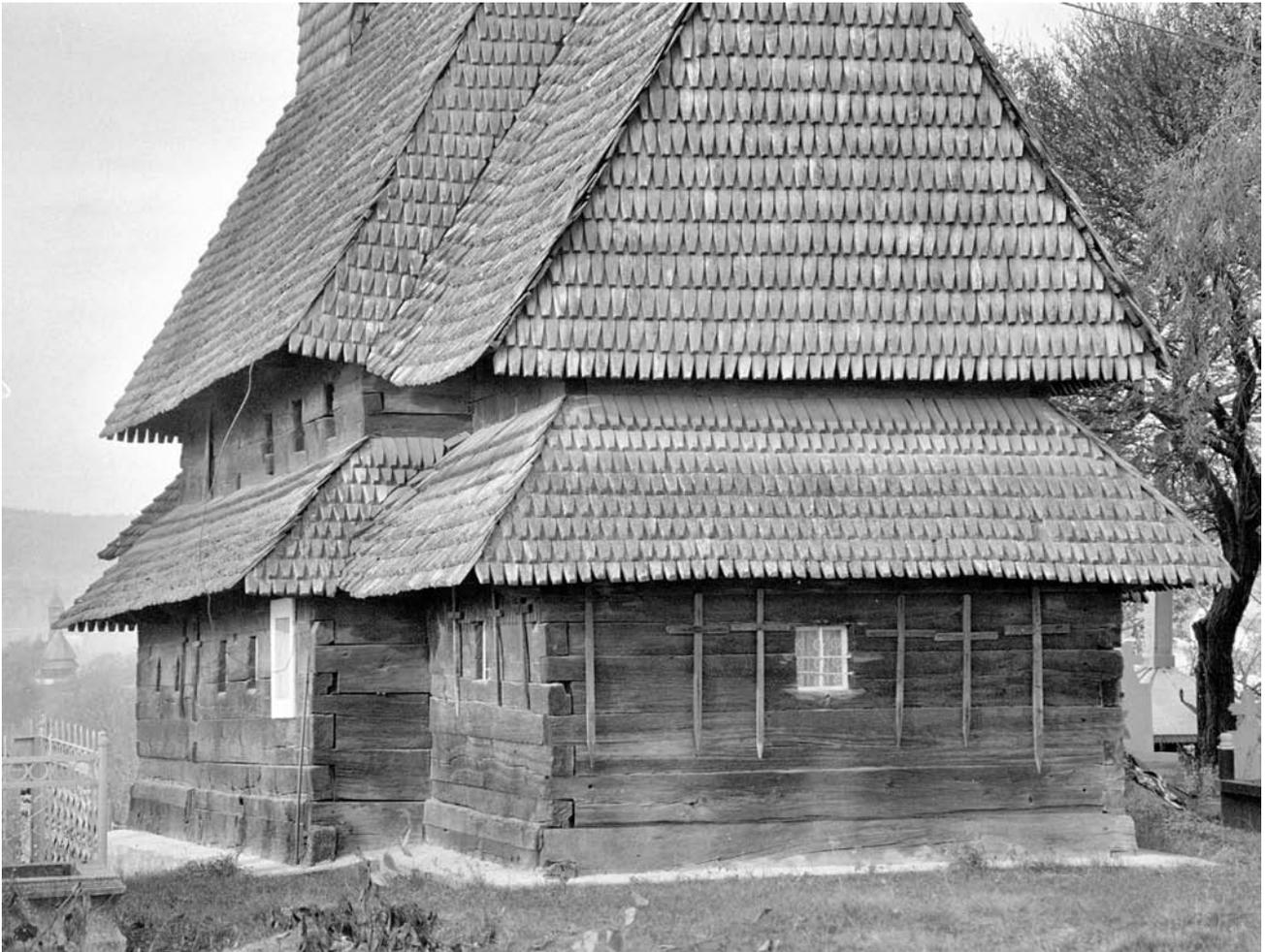
45 *Apşa de Mijloc Susani*. This medium sized wooden church, from the first decade of the 18th century, was excellently built with well levelled walls and flush covert joints. Photo: October 2000.
