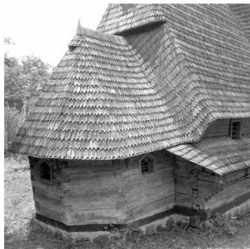
**46** *Corneşti*. The sanctuary, erected in the first decade of the 16th century, displays well refined covert joints and a higher quality of wood work than the rest of the church (finished probably in 1615 and significantly repaired in the 1670s). The local oral tradition indicates the origin of the sanctuary from the Iza Valley. Scale drawing of the rear from August 1997, of a joint from June 1998 and photo from June 1996.
