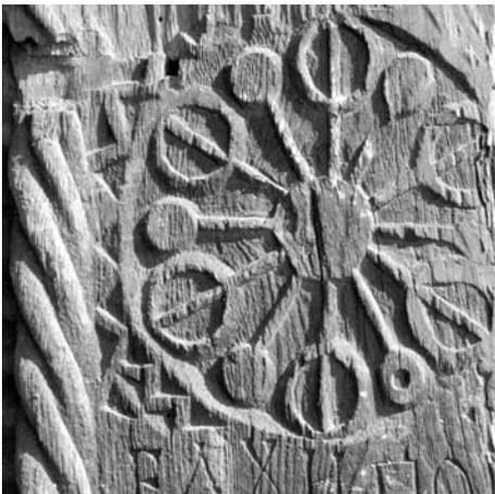
**148** *Budeşti Josani*. Detail from the portal of the entrance. The rosette motive was cut in a bas-relief technique while the lateral moulding in relief from the same piece of jamb. Photo: June 1999.
