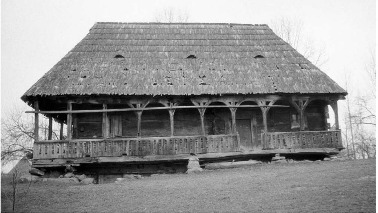
**29 Sârbi.** The manor house of the noble Dunca de Sârbi family (1690s). The corner joints present a small recess in the neck to improve the interlocking of the beams (below, left). Due to the limited length of the massive logs the house was extended lengthwise by posts, one of them also used as the left jamb of the entrance (below, right). Photos: March 1995, on the initial site (above and below), and August 1997, during its reconstruction in the Maramureş Museum.
