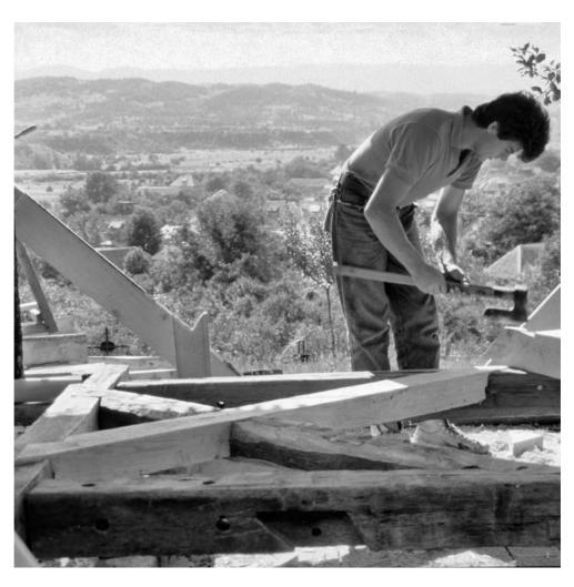
**132** *Bârsana.* The work with a tower frame required a plane place where the pieces were cut and marked to be reassembled above the church. Here a carpenter cut a new cross brace for the tower of the former monastery church of Bârsana during the last repairs. Photo: July 1997.
