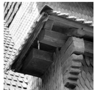
**154** *Nyzhnie Selyshche*. The serrated consoles with slightly rounded edges were specific for the oldest churches of this itinerary. Photo from Blansko, Czech Republic: April 1997.
