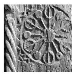
**148** *Budești Josani.* Detail from the portal of the entrance. The rosette motive was cut in a bas-relief technique while the lateral moulding in relief from the same piece of jamb. Photo: June 1999.
