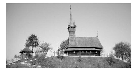
**125** *Apşa din Jos.* The heavy bells were moved from the massive tower and housed in the lower but secure belfry in front of it. Photo: October 2000.
