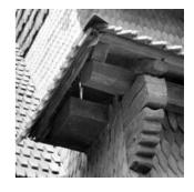
**154** *Nyzhnie Selyshche.* The serrated consoles with slightly rounded edges were specific for the oldest churches of this itinerary. Photo from Blansko, Czech Republic: April 1997.
