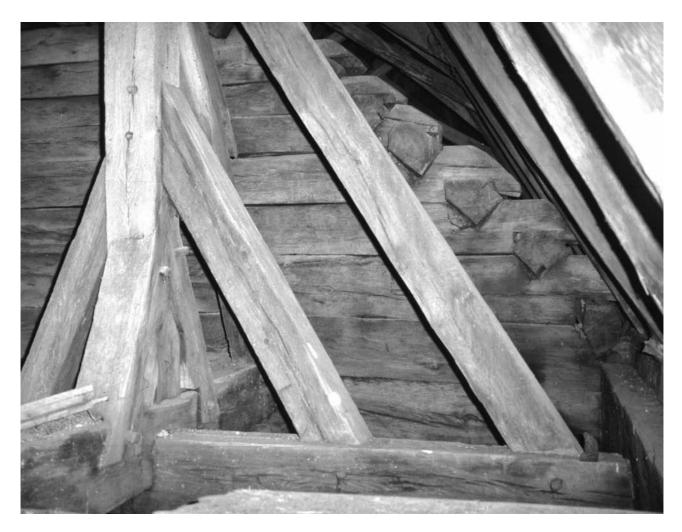
**127** *Apşa din Jos.* The anchoring of the south-eastern upright in the massive transoms of the base. The transoms were interlocked with the lateral walls while the log fabric was still in construction assuring a stable connection between them. Photo: October 2000.
