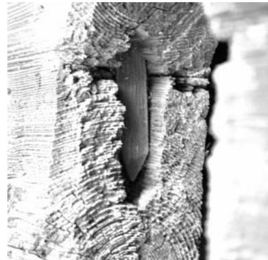
60 Botiza. The scratched line marking the position of the dowel before drilling was still visible after 4 centuries. Photo: October 2001
