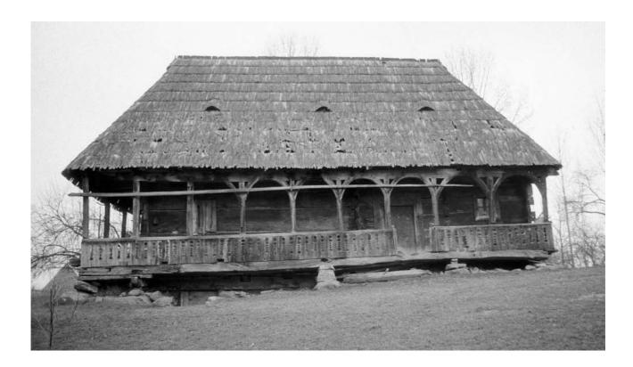
*Sârbi*. The manor house of the noble Dunca de Sârbi family (1690s). The corner joints present a small recess in the neck to improve the interlocking of the beams (below, left). Due to the limited length of the massive logs the house was extended lengthwise by posts, one of them also used as the left jamb of the entrance (below, right). Photos: March 1995, on the initial site (above and below), and August 1997, during its reconstruction in the Maramureş Museum.
