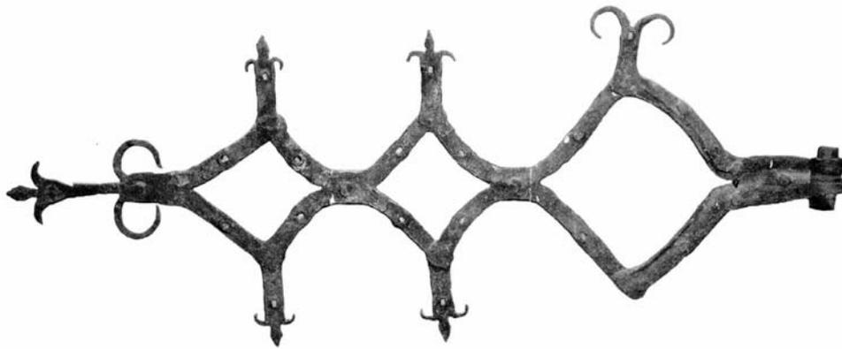
70 Ieud Șes. The decorative iron hinges of the inner door to the nave (below) remind of the surviving hinge from the inner door in the church of Dragomirești (above) indicating the work of a single smith behind both. The two close churches were also built soon one after the other in the 1710s. Photos: July 1997 (below) and June 1999 (above).
