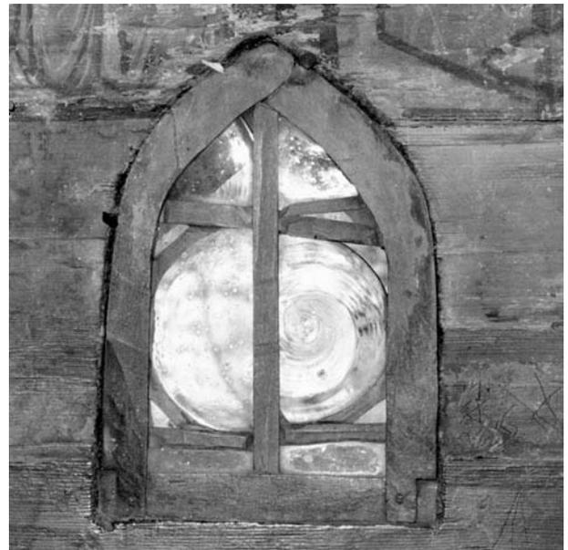
wooden nails into a groove following the aperture in the wall. The bottle glasses, for the most part used in small shivers, were embedded in the frame by delicate grooved pieces of sycamore maple wood. Until the end of the 18th century, the majority of the churches were supplied with such windows.
