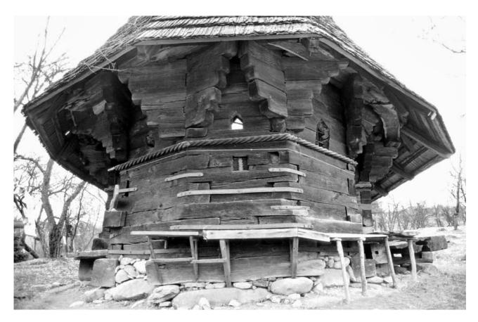
**175** *Sârbi Susani*. The rear of the sanctuary with the joyful play of consoles under the eaves. The only original window seems to have been the square one bellow the moulding rope. The rope appears to have separated the earthly world from the heavenly one. Photo: Spring 1995.
