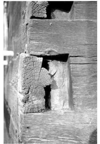
48 *Breb*. Settings in the north-western corner of the building damaged the hook in the picture exposing the covert cog. However, the damage was limited thanks to the presence of the heart of the tree in the hook. The visible traces indicate the cog was cut with an axe. Photo: October 2000.
