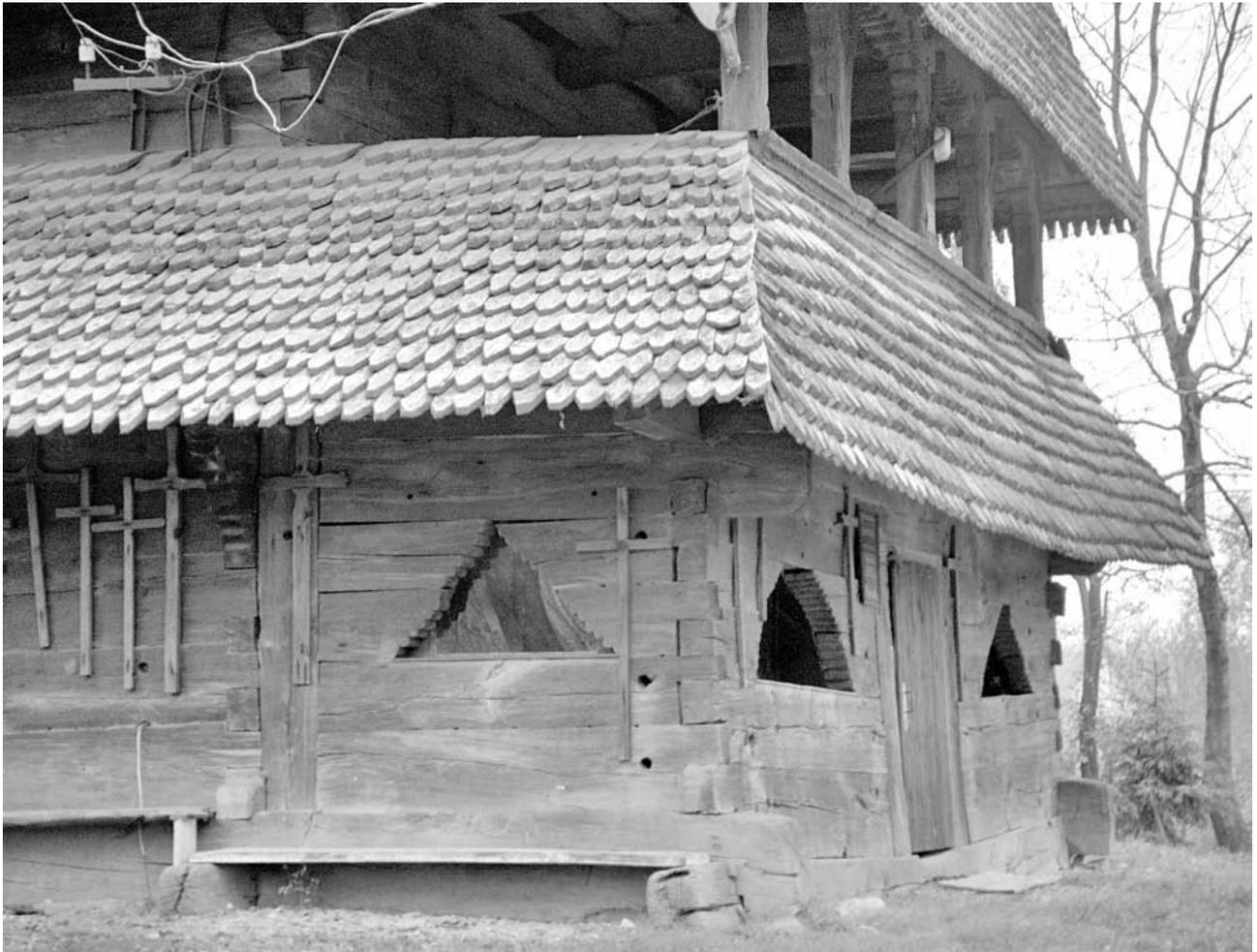
**157** *Sokyrnytsia*. The porch on two levels, an open loggia above and a massive walled antechurch at the level of the entrance. Photo: October 2000.
