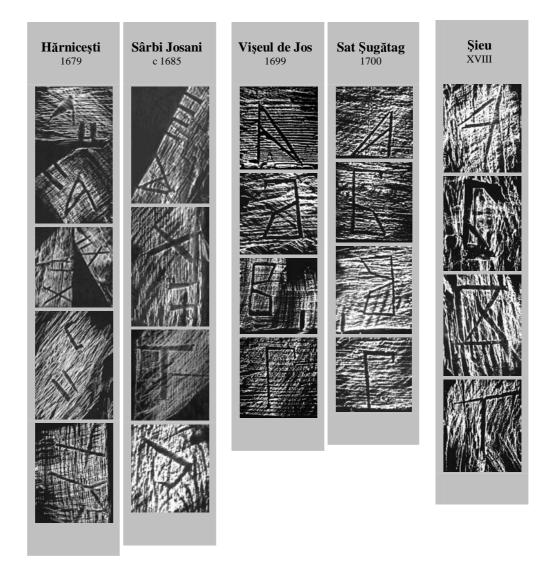
*Mixed assembly marks from the 16th, 17th and 18th centuries.* The Cyrillic signs were most often mixed with other types of signs. These are only a small number of the existing ones in the respective tower frames, mainly from around the base, where they are easier to reach. Tracing: October 2000 and 2001.
