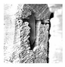
**60** Botiza. The scratched line marking the position of the dowel before drilling was still visible after 4 centuries. Photo: October 2001
