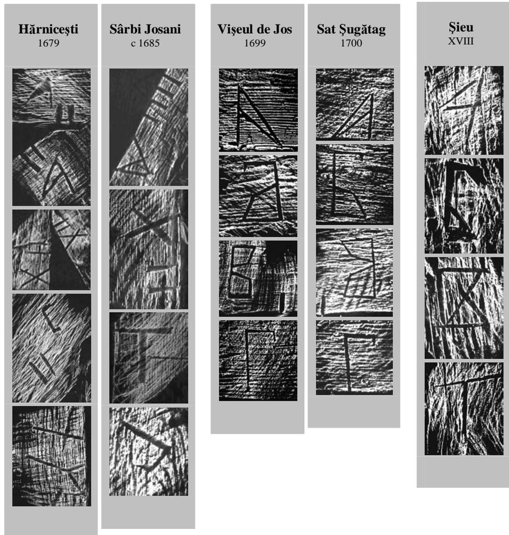
**135 Mixed assembly marks from the 16th, 17th and 18th centuries.** The Cyrillic signs were most often mixed with other types of signs. These are only a small number of the existing ones in the respective tower frames, mainly from around the base, where they are easier to reach. Tracing: October 2000 and 2001.
