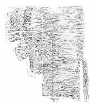
**159** *Sokyrnytsia.* The church carpenter liked to round off the serrated profile of the consoles. The working lines are still traceable on one of them. Tracing at the scale 1:4, July 1998.
