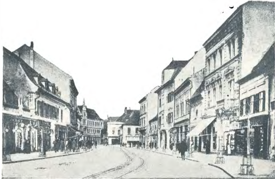
Strada Heltan. — Heltan Strasse. — Rue Heltan.
